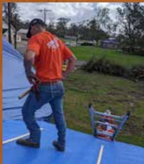
Jayme Baker targs a roof to prevent further storm damage.
